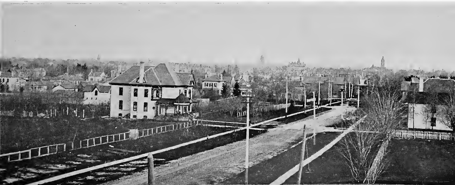
VIEW FROM ST. JAMES STREET, LOOKING SOUTH.
