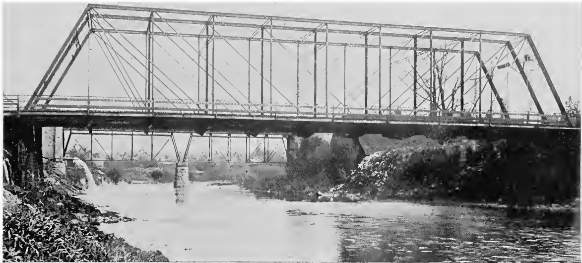
YORK STREET (WESTMINSTER) BRIDGE.
