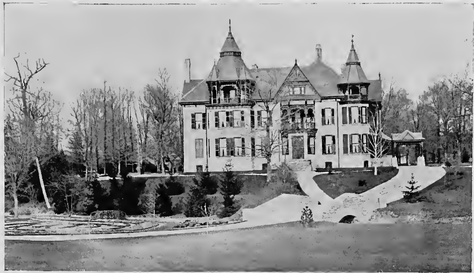
"WAVERLEY," RESIDENCE OF T. H. SMALLMAN.
