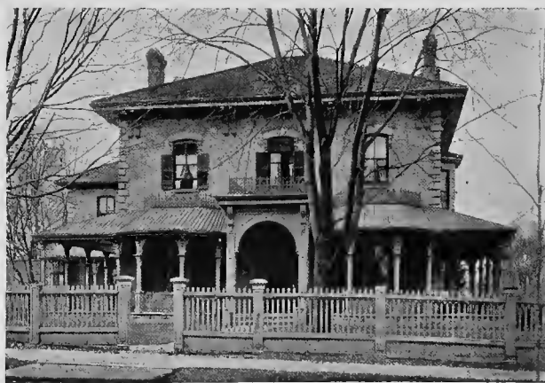
RESIDENCE OF T. H. CARLING.
