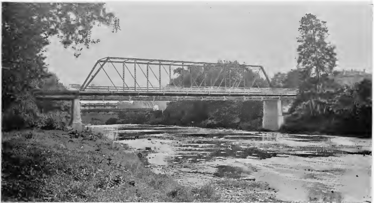
KING STREET BRIDGE, CARRYING TRUNK SEWER.
