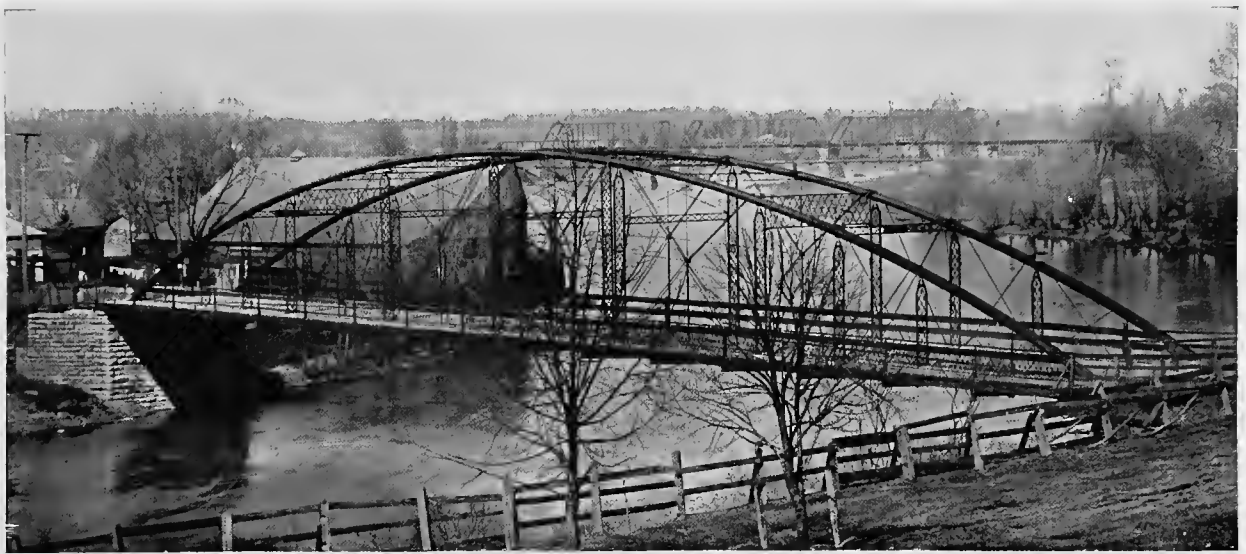
BLACKFRIARS, OXFORD, AND C. P. R. BRIDGES.
