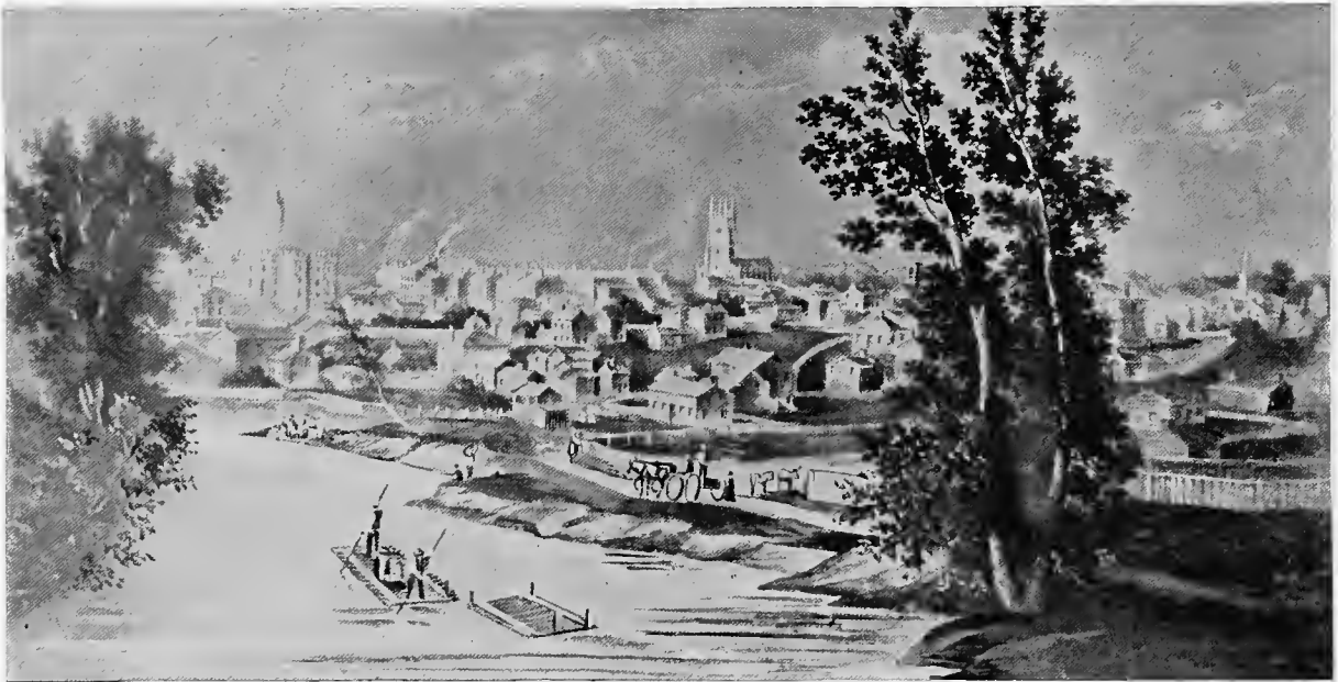
VIEW OF THE SOUTHERN PART OF CITY WHILE GRADING FOR THE G. W. R.
