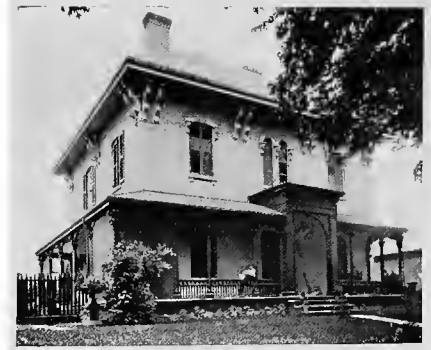
RESIDENCE OF T. F. KINGSMILL.
