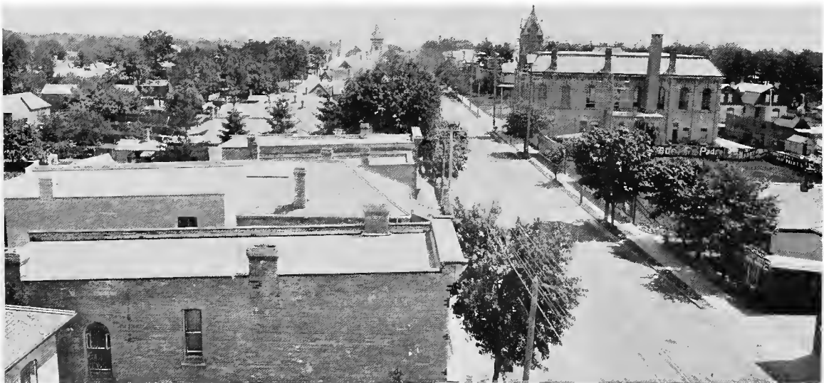
VIEW, LOOKING EAST, SHOWING EASTERN FIRE HALL NO. 2.
