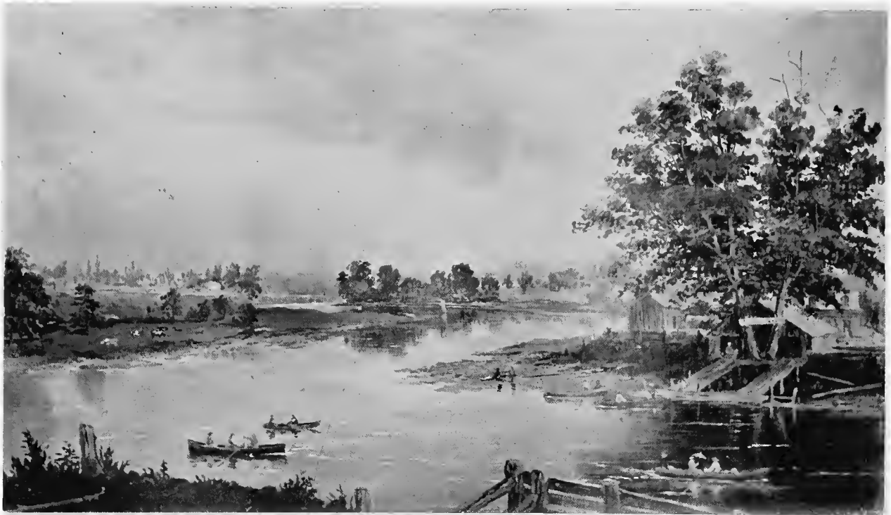
VIEW FROM FOOT OF DUNDAS STREET, LOOKING WEST, 1875.
