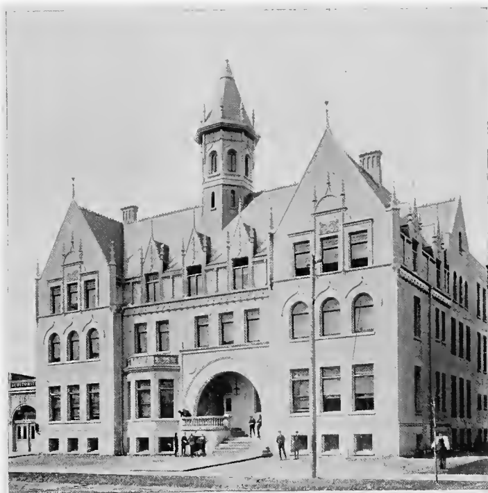
YOUNG MEN'S CHRISTIAN ASSOCIATION BUILDING. Wellington street.
