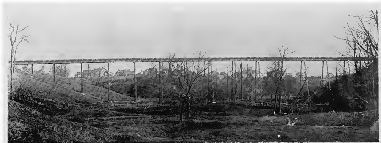
MILL CREEK BRIDGE, ON L. E. & D. R. RAILWAY — LENGTH 547 FEET 8 INCHES, HEIGHT 76 FEET.
