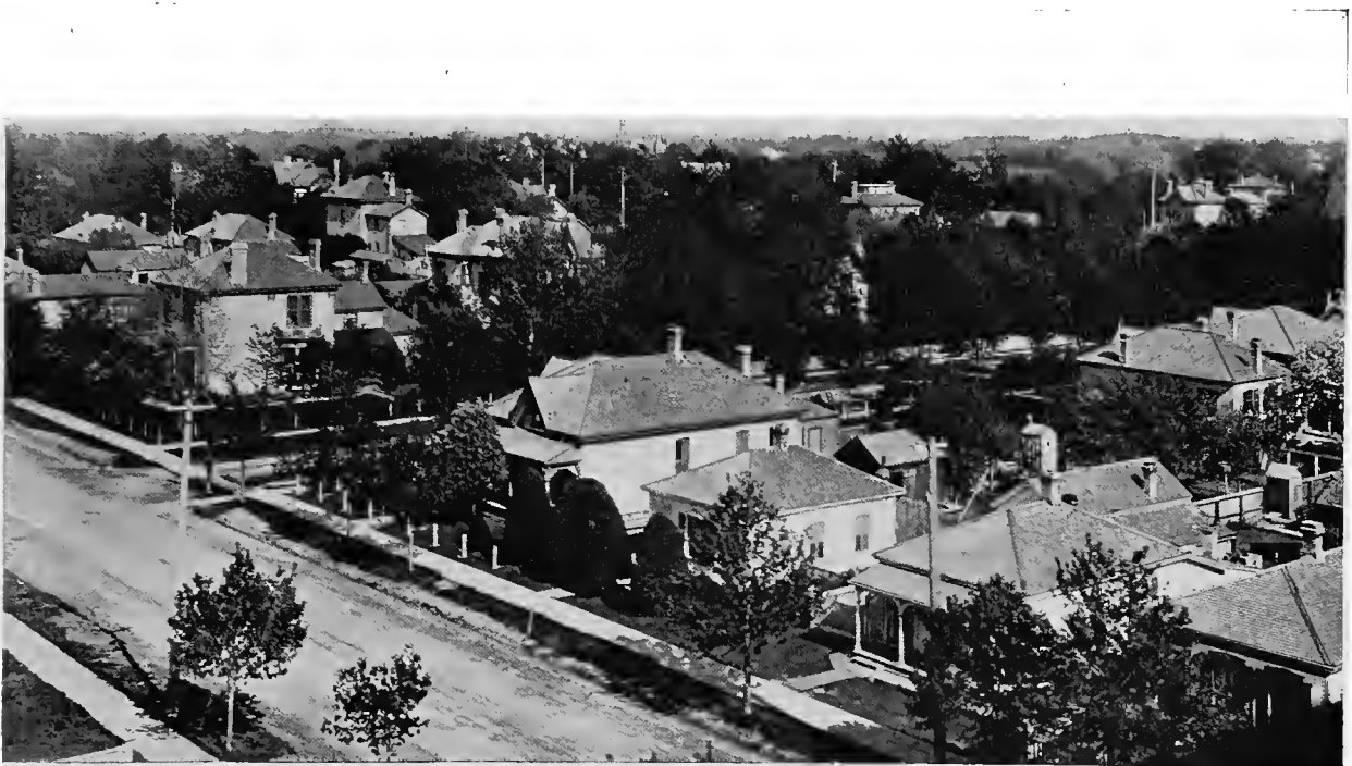
VIEW, LOOKING SOUTH-EAST FROM SOUTHERN FIRE HALL NO. 3.
