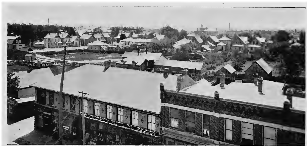
VIEW, LOOKING SOUTH-WEST FROM NO. 2 FIRE HALL.
