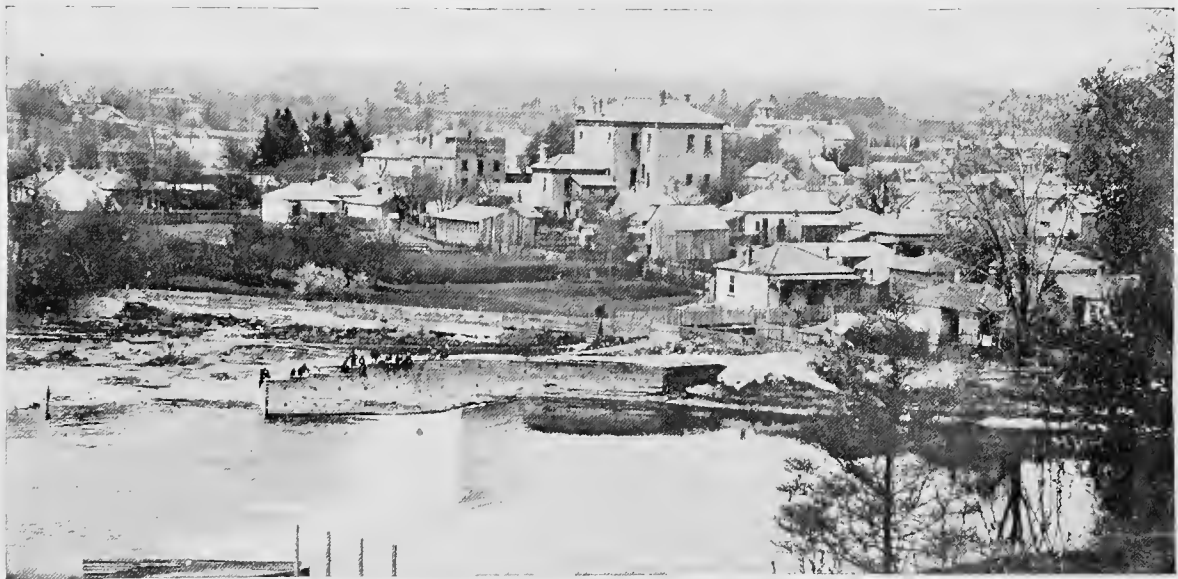
A PORTION OF NO. 2 WARD, FORMERLY LONDON WEST, FROM KENT STREET.
