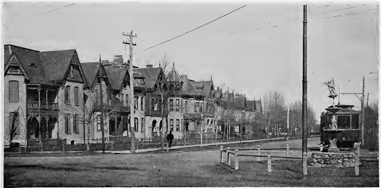
CENTRAL AVENUE, NORTH OF VICTORIA PARK, LOOKING EAST FROM RICHMOND STREET.
