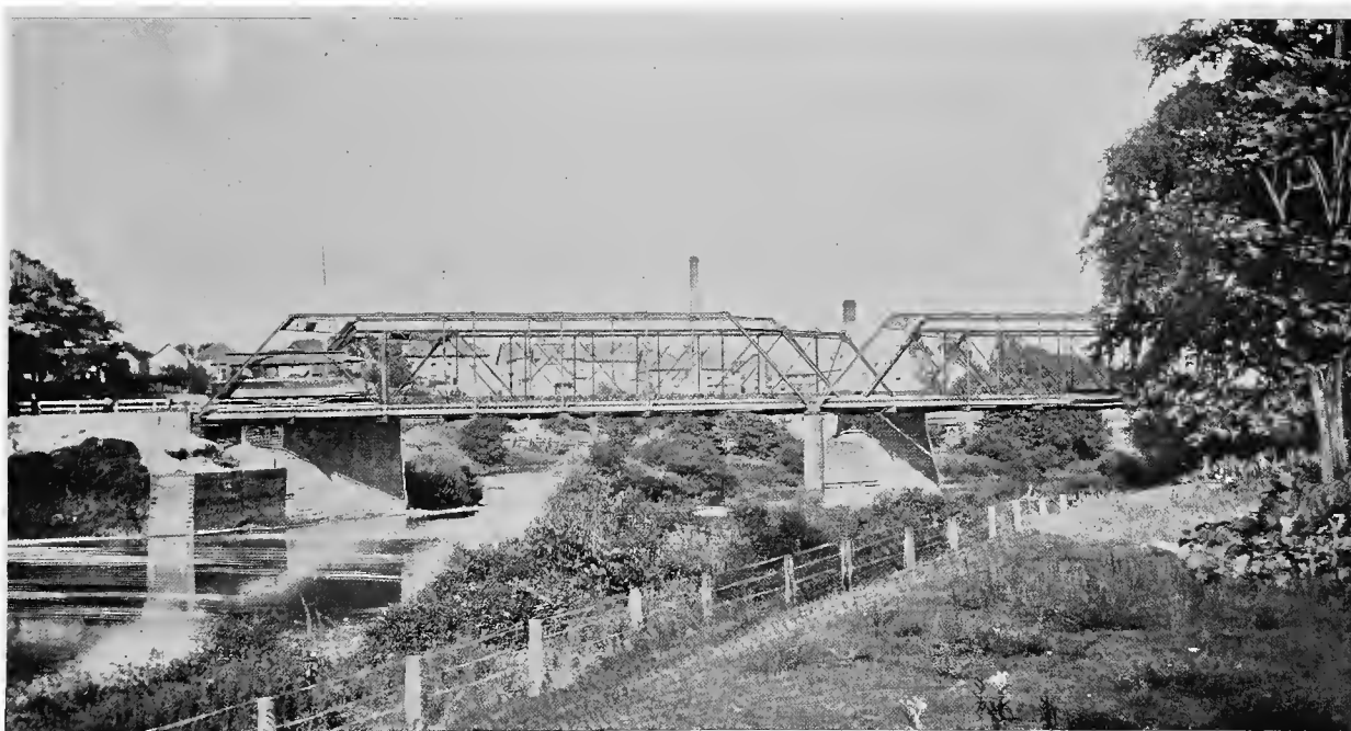
VICTORIA BRIDGE, RIDOUT STREET SOUTH.
