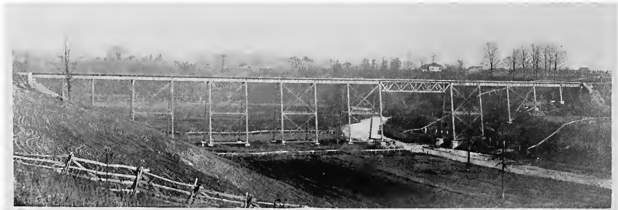
KETTLE CREEK BRIDGE, ON L. E. & D. R. RAILWAY — LENGTH 613 FEET, HEIGHT 73 FEET.
