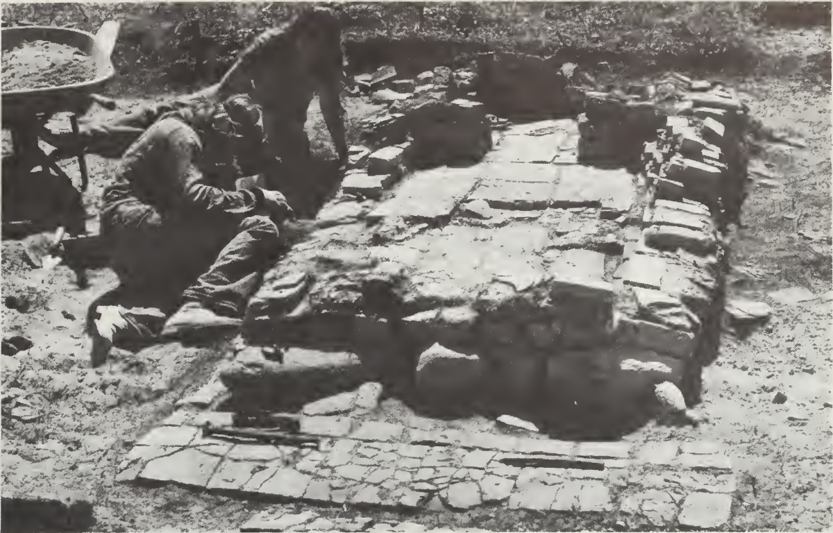
Plate 148 Base of a stove, Charlton Island.
