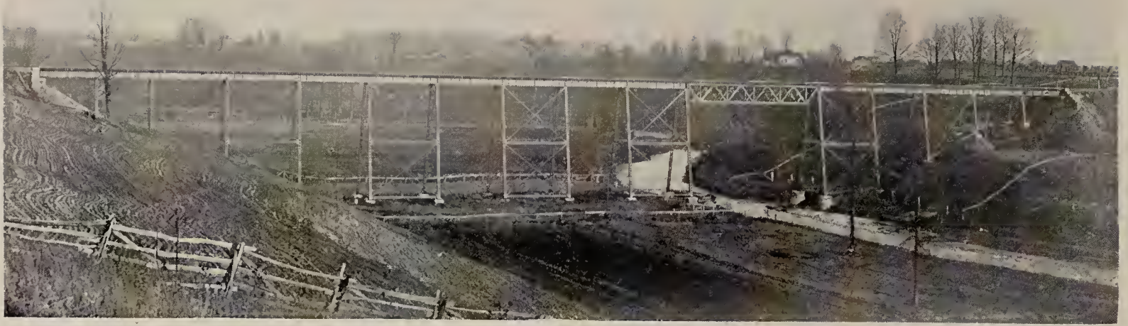
KETTLE CREEK BRIDGE ON L. E. & D. R. R. — LENGTH 613 FEET, HEIGHT 73 FEET.
