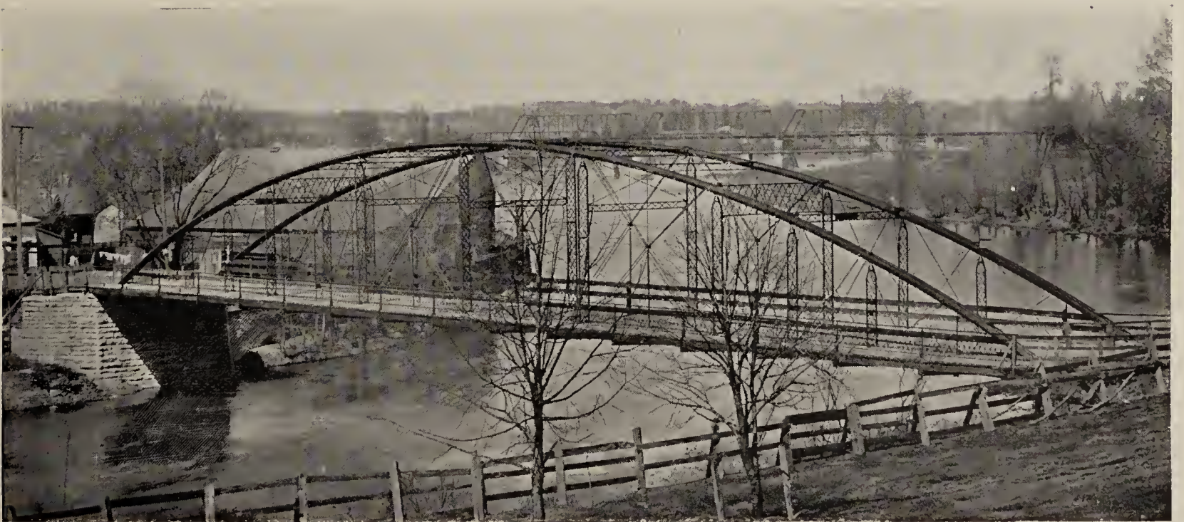
BLACKFRIARS, OXFORD, AND C. P. R. BRIDGES.
