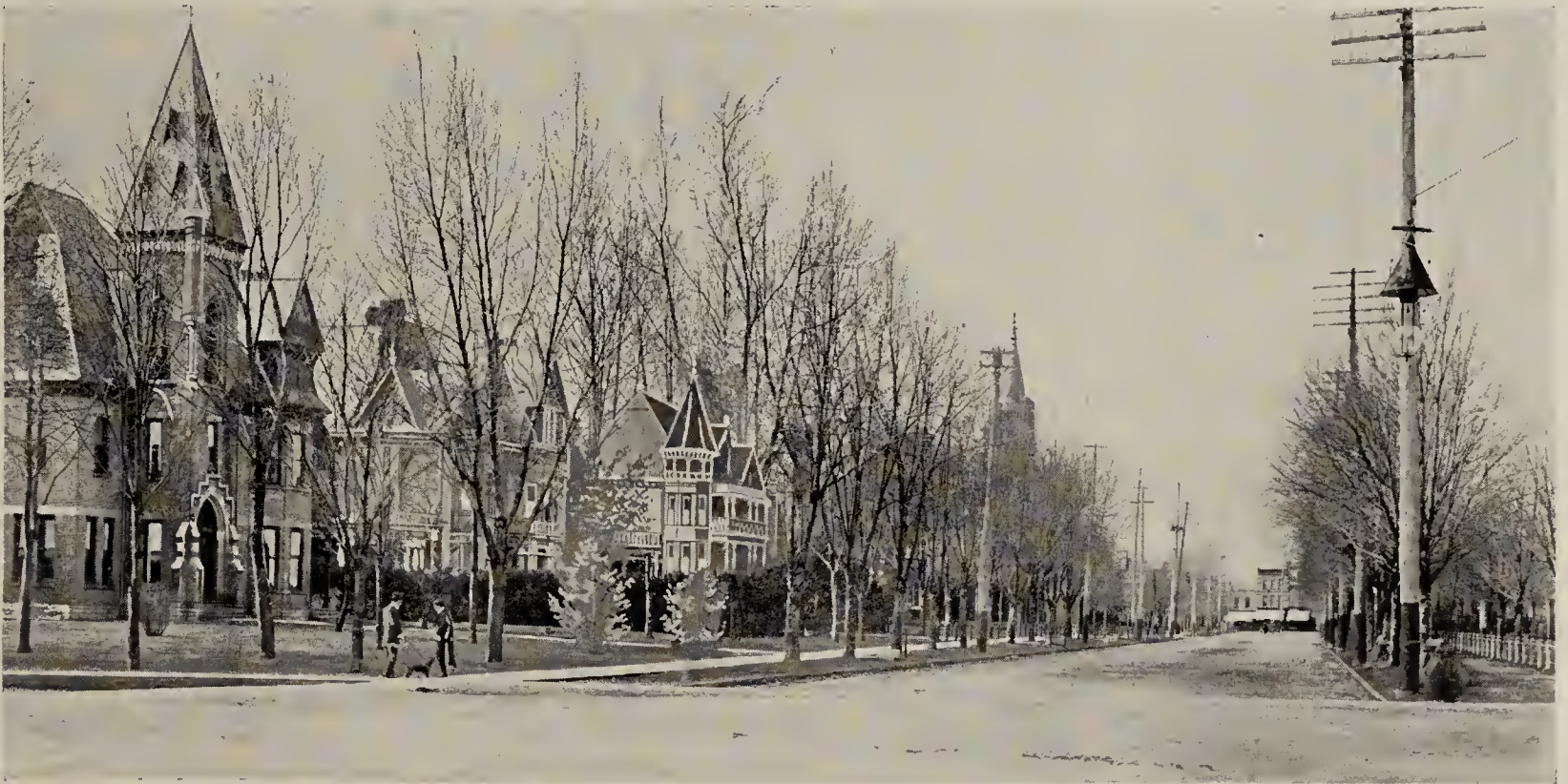
DUFFERIN AVENUE, SOUTH OF VICTORIA PARK, LOOKING WEST FROM WELLINGTON STREET.
