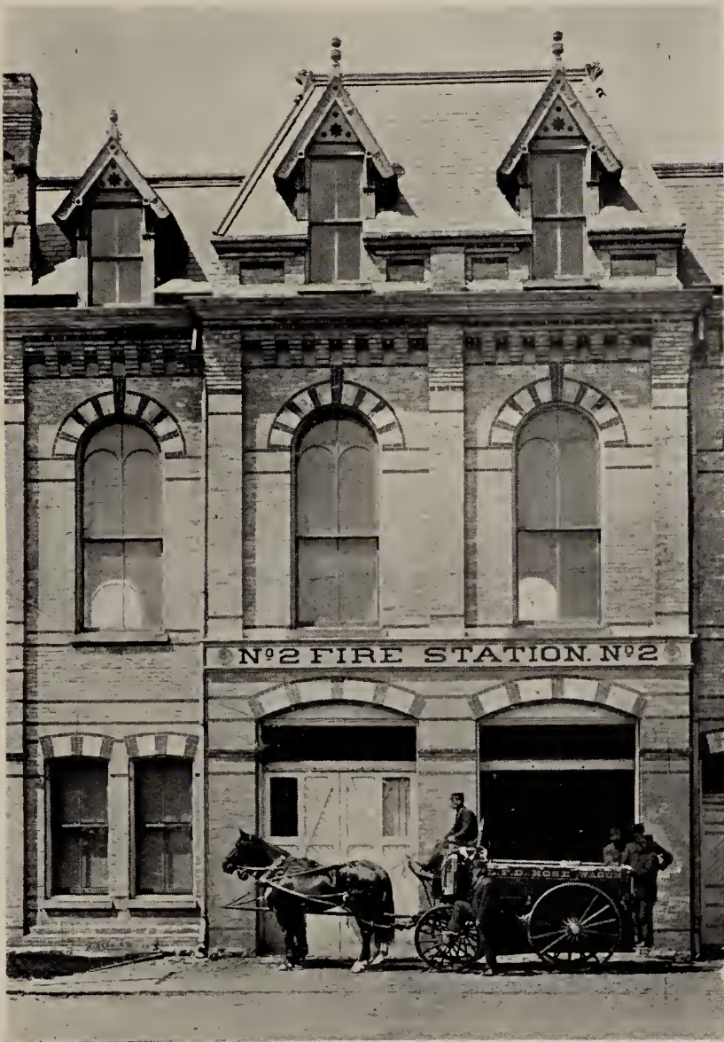
NO. 2 FIRE STATION.
