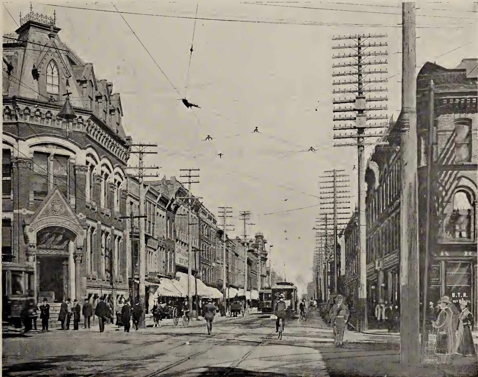
DUNDAS STREET, LOOKING EAST FROM RICHMOND.
