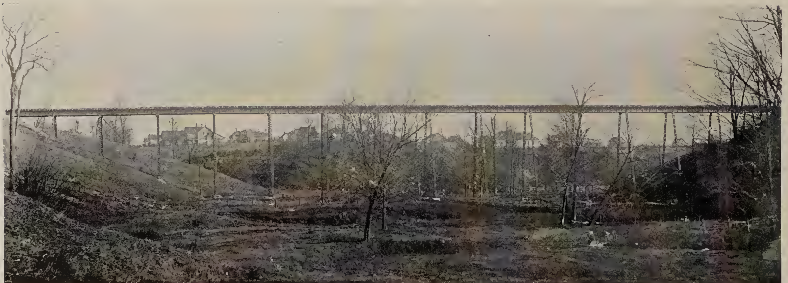
MILL CREEK BRIDGE ON L. E. & D. R. R. — LENGTH 547 FEET 8 INCHES, HEIGHT 76 FEET.
