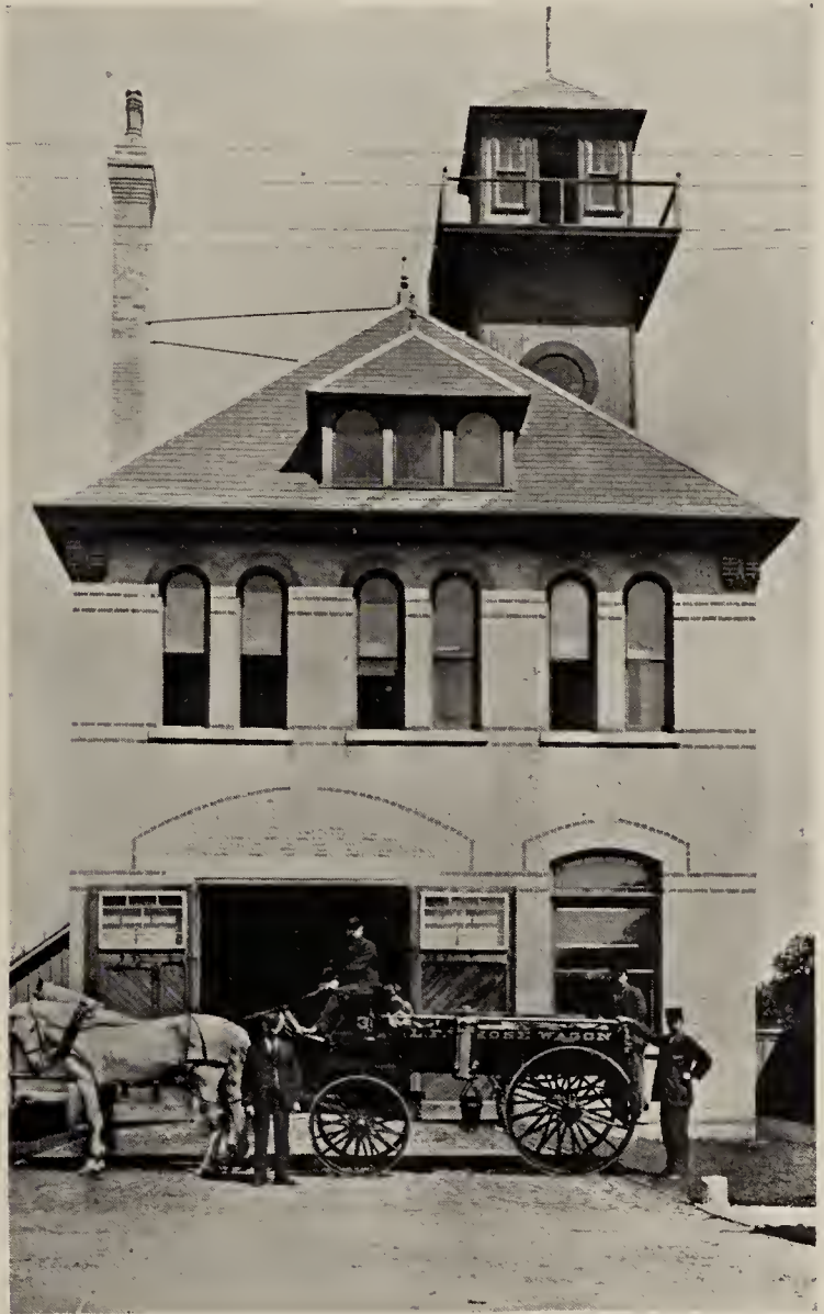
NO. 3 FIRE STATION.
