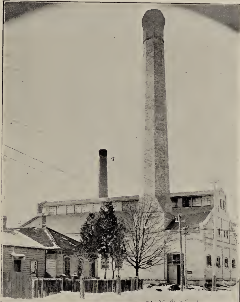
LONDON STREET RAILWAY POWER HOUSE.
