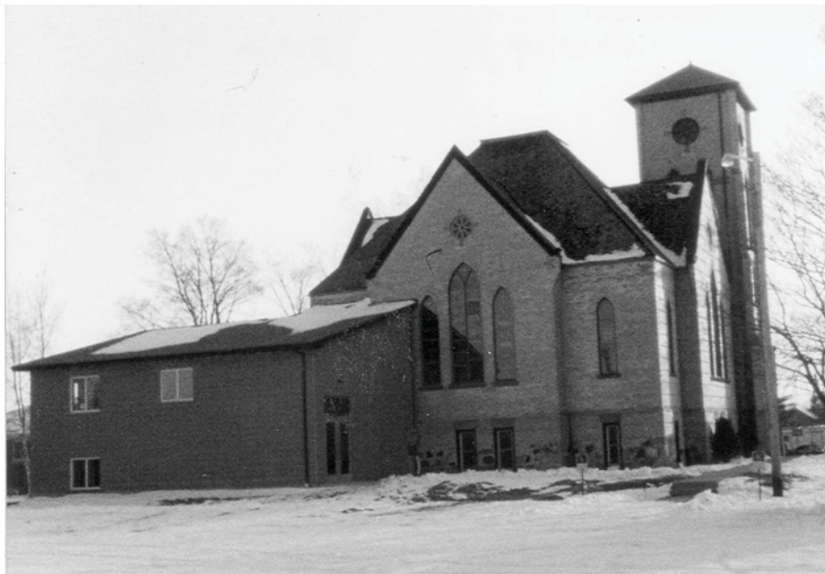
Views of completed addition on December 14 th 1992
