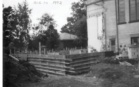
Old part just about removed
