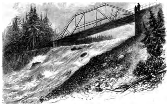
ROCKY RIVER BRIDGE.
