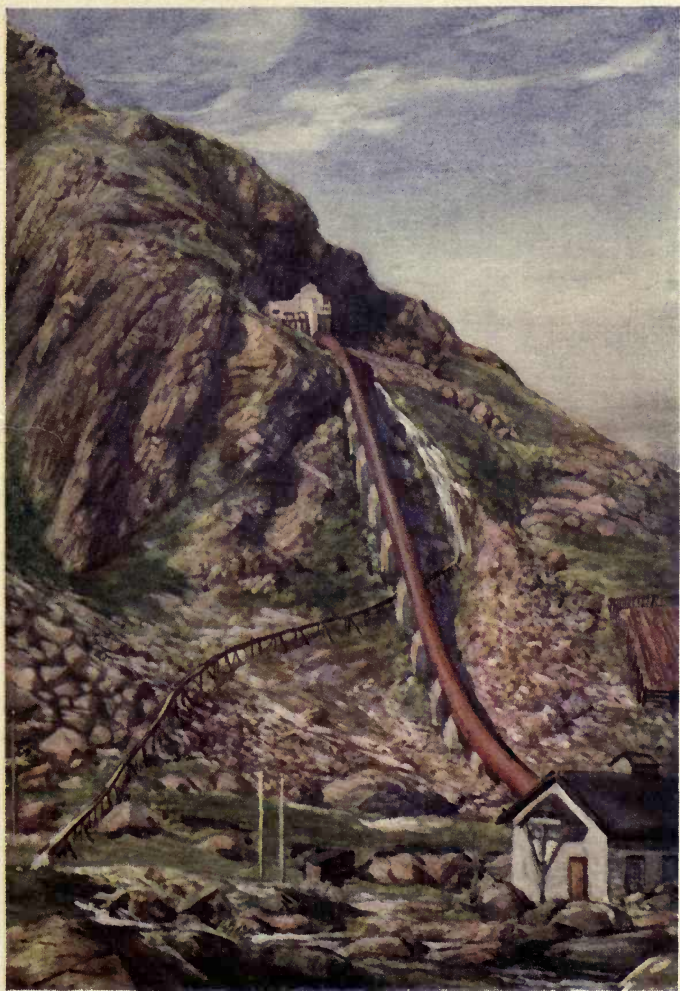
THE WATER "FLUME" AT PETTY HARBOUR, WHERE ELECTRIC POWER FOR ST. JOHN'S IS GENERATED.
