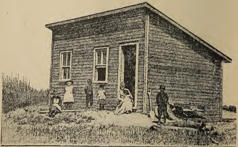
No. 4.—Cost $120 (£24).—This house has one room, 18 × 12 ft., cellar underneath, with trap door in floor.
