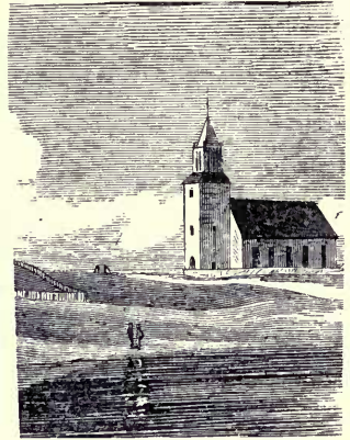
Church at St. Andrew's Rapids Dedicated May 1st, 1832
