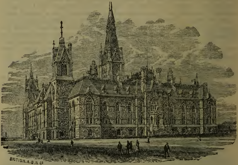
BRITISH A. S. N. C. DEPARTMENTAL BUILDINGS, OTTAWA.—WEST BLOCK.
