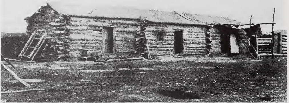
Figure 6a. "Half-breed" house, Wood Mountain Settlement, Saskatchewan. This is a typical house used in areas occupied by the peoples of the Lower Saskatchewan south of the fertile belt. Successive extensions, forming a multiple-dwelling unit, are known to have been employed at St. Albert prior to the smallpox of 1870. St. Albert houses, however, used post-on-sill construction with logs squared by broad-axe. National Archives of Canada, C-81781, 1975-122 (G. M. Dawson, Case 42, No. 169, Album 2, p. 45).
