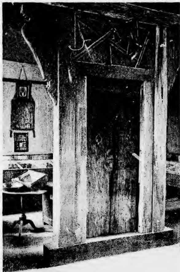
The Door of the Old Indian House
