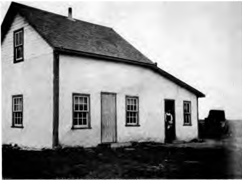
Type of average house, File Hills Colony, showing kitchen which serves first years until money is made from crops to build main structure.
