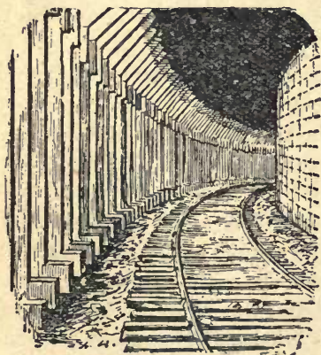
A SNOW-SHED ON THE C. P. R.
