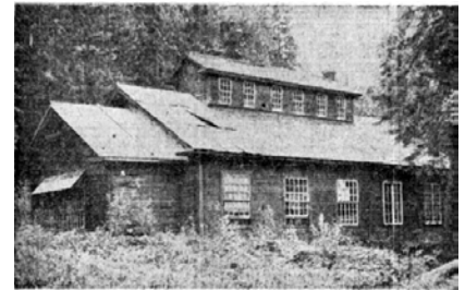
Kaslo powerhouse. Touchstones Nelson
