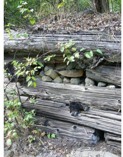
Cribbing on the Kaslo dam. Touchstones Nelson
