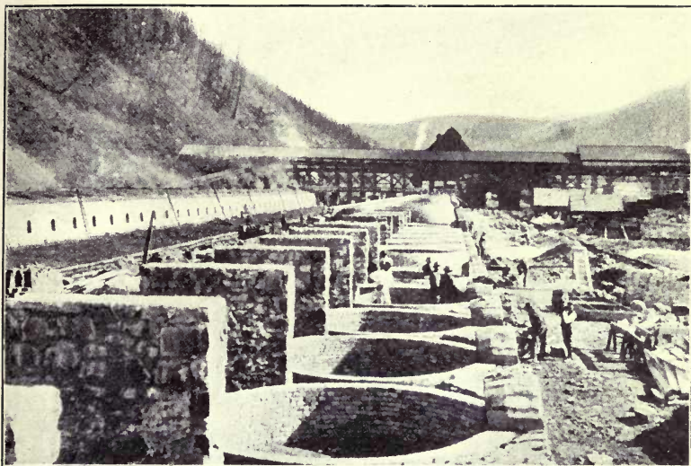
CROW'S NEST PASS COLLIERIES—TIPPLE AND COKE OVENS AT MICHEL, B.C. Showing Ovens in operation and others in course of building.
