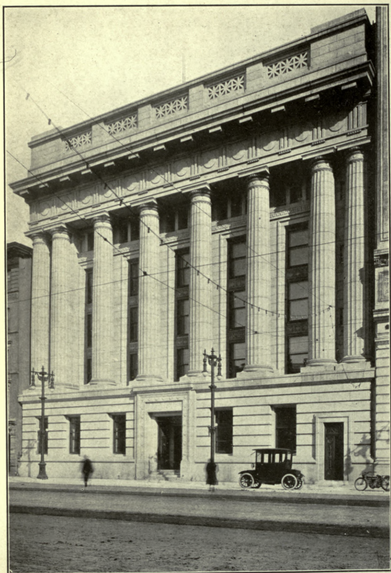
THE NEW CANADIAN BANK OF COMMERCE BUILDING AT WINNIPEG, 1912.
