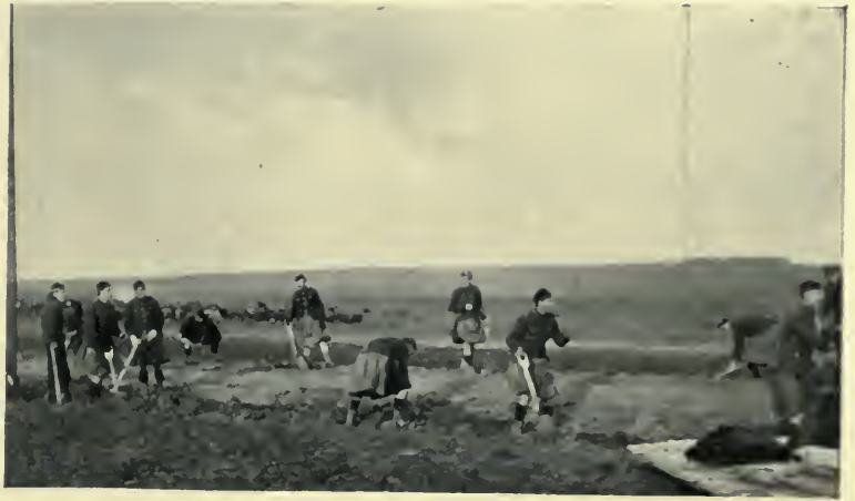
DIGGING TRENCHES—SALISBURY PLAIN.
