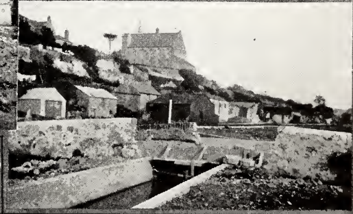
NEW WAY BRIDGE - RECONSTRUCTION
