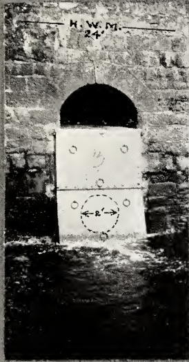
THE VALVES THAT DID THE TRICK HALF-TIDE - RISING - LOWER VALVE STILL WORKING (N.B. ARCH ON OUTER FACE IS HIGHER THAN ARCH OF CULVERT. THE DOTTED CIRCLE SHOWS CLEAR SECTION OF OLD VALVE FOR COMPARISON.
