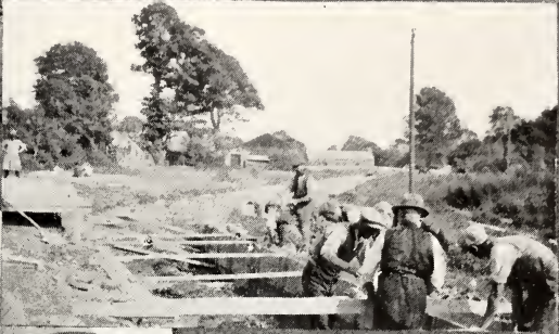
THE BEND AT ROCK TERRACE FIXING SHUTTERING
