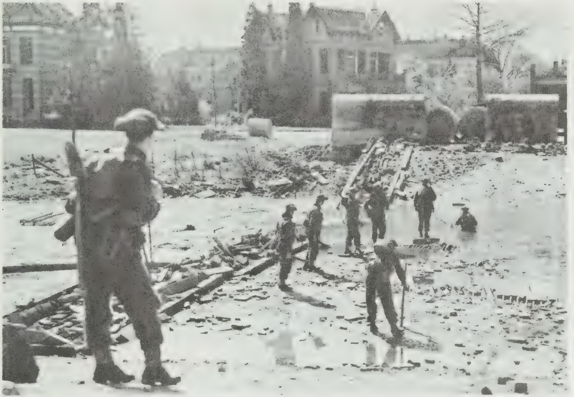
North Shore Regiment "C" Coy crossing the canal at Zutphen, 7 April 1945. (Public Archives Canada 49399)
