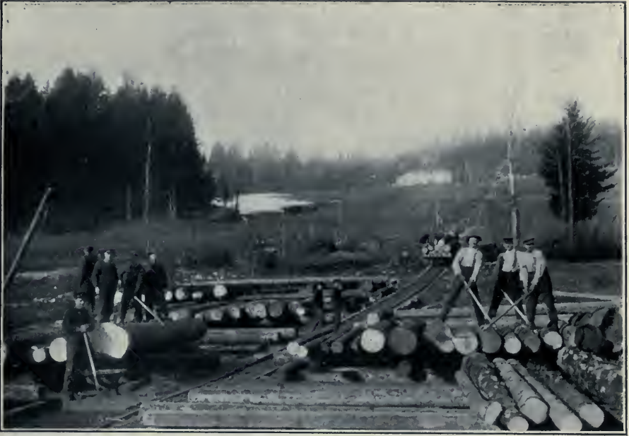
No. 44. Railing Logs : Part of a 2,000 ft. Track which drops 195 ft.
