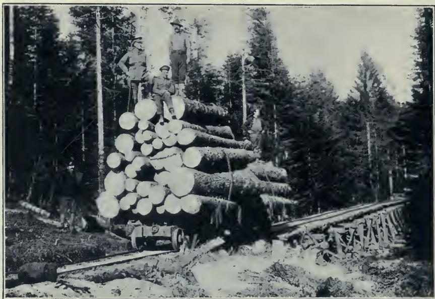
No. 33. Truck-load at the end of a 600 ft. Trestle in the Vosges.
