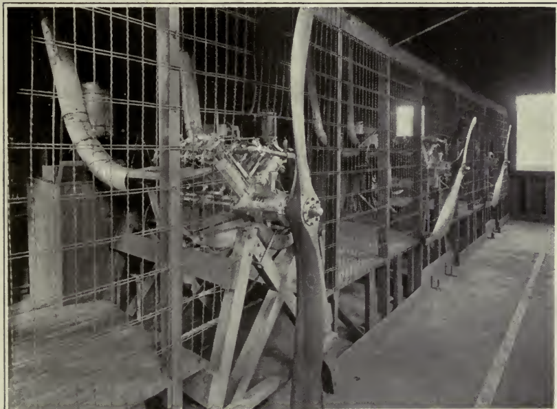
THE STARTING END. (NOTE PROTECTIVE SCREEN).
