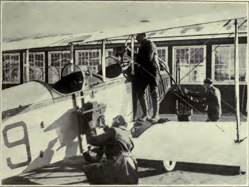
ATTACHING CAMERA TO FUSELAGE.
