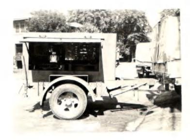
The function of this equipment is to supply 100-volt direct current for the operation of high current density carbon are searchlights.
