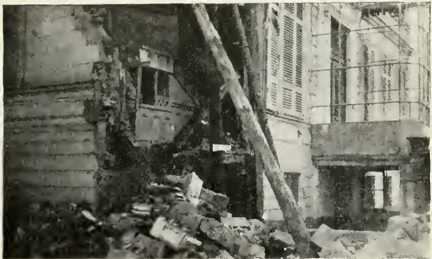
CONTROL PIT, ST. SAULVE.
