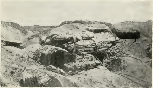
CONTROL PIT, ROCLINCOURT.
