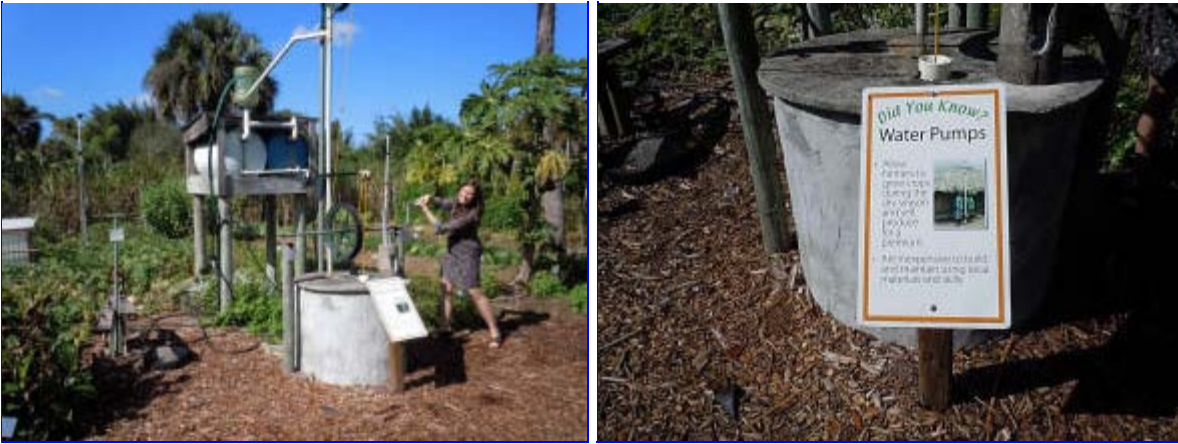
Low Tech Water Pump & Storage
